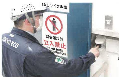
入室制限 (IC カード + 指静脈認証) Room access control (IC card + finger vein authentication)
