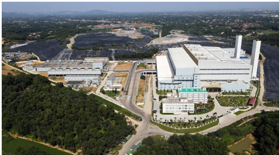
Soc Son Waste-to-Energy Plant
