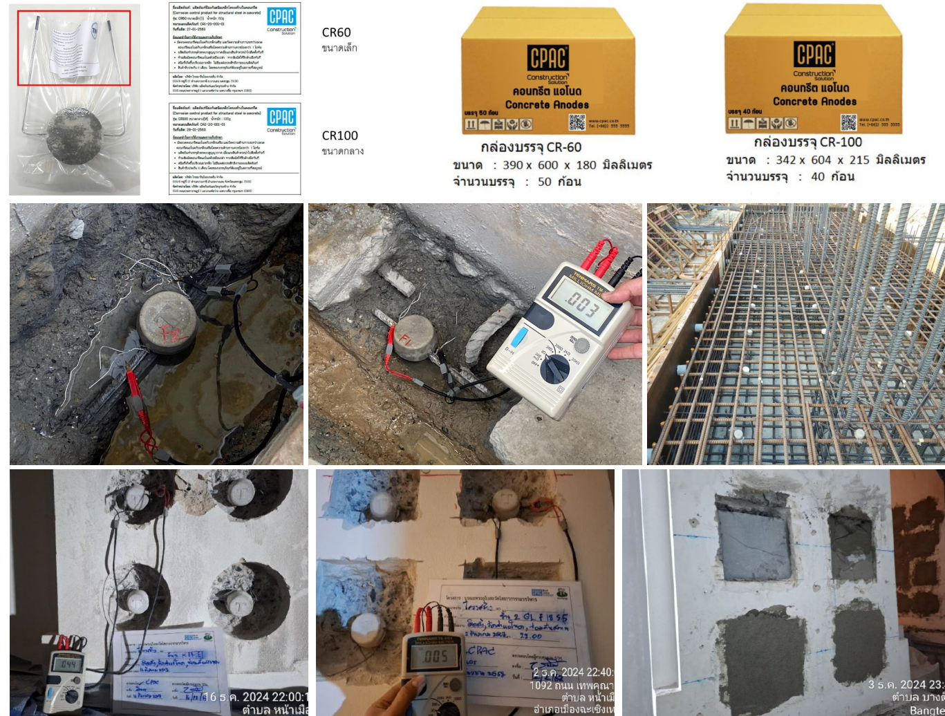
Installing Concrete Anode for Protecting Rebars inside Concrete Structures
