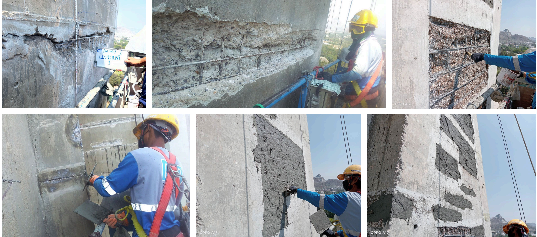
Repairing Processes with Patching Method
