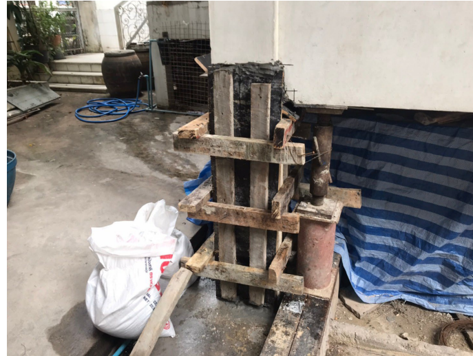
Repairing Processes with Grouting Method (Column)
